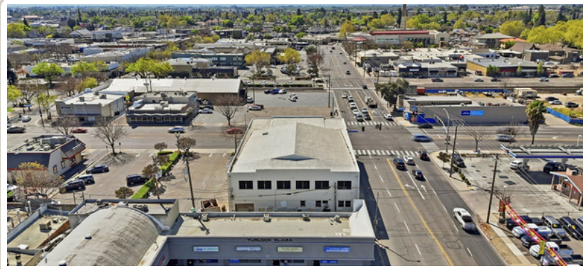
Olive Ave frontage and adjacent parking
