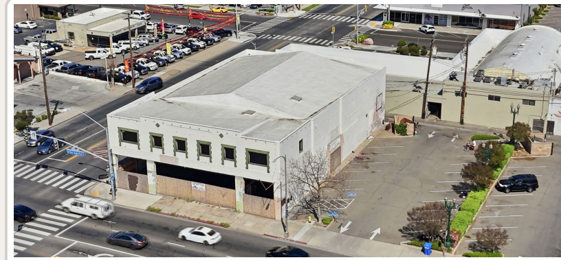
Existing condition from easterly angle
