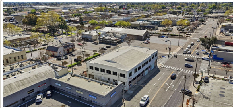
Street-level front corner presence
