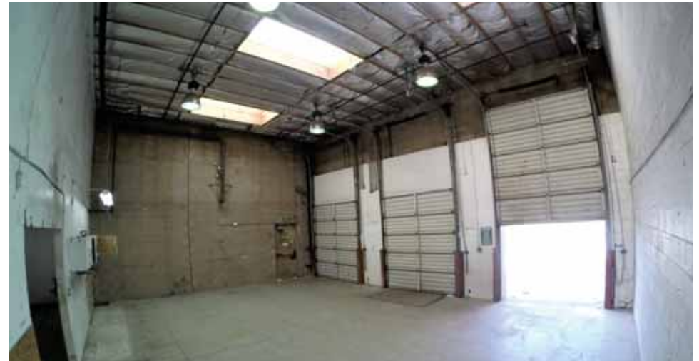
Receiving Area Dock High Roll Up Doors 8' W x 9' H
