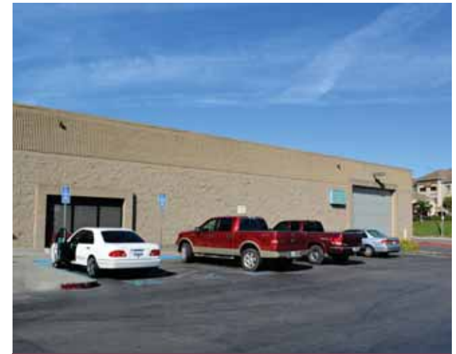
Customer Pick Up Entrance - 20' W x 15' H Roll Up Door
