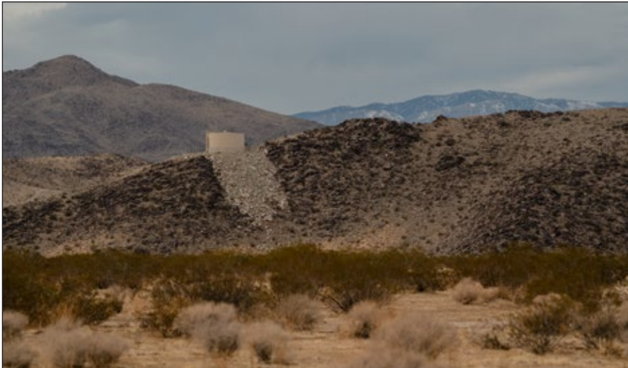
Facing West | Water Tank In Background
