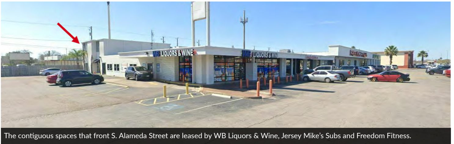
The Morningside Shopping Center office space facing Gordon Street (510 Gordon Street) is included in this offering.
