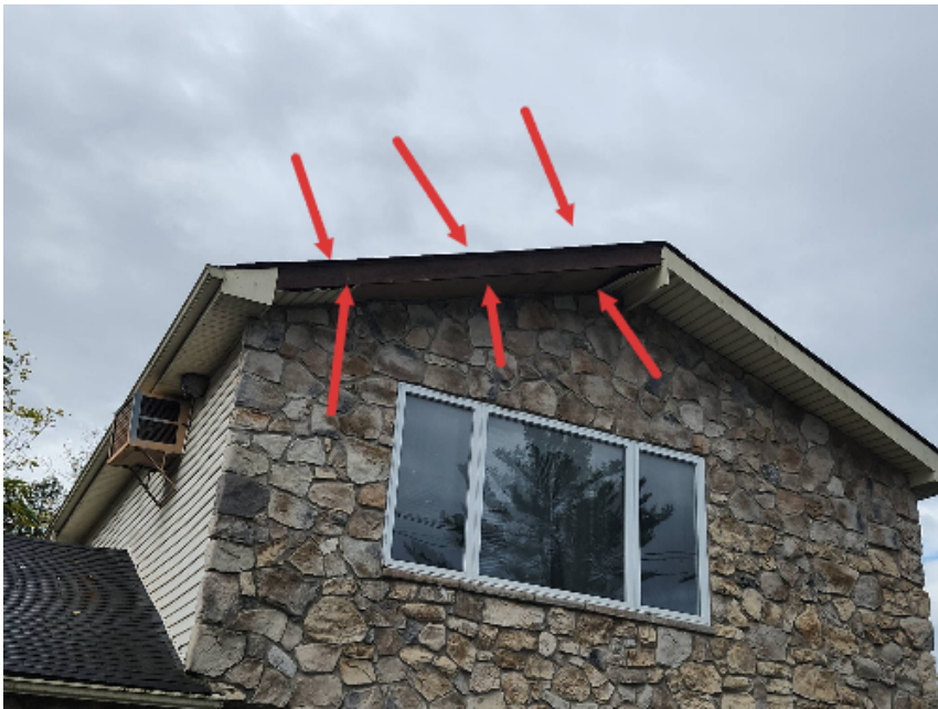
Missing soffit and fascia
