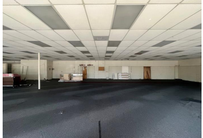
Current condition of interior
