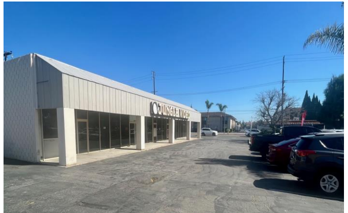
View looking towards Edinger Ave access
