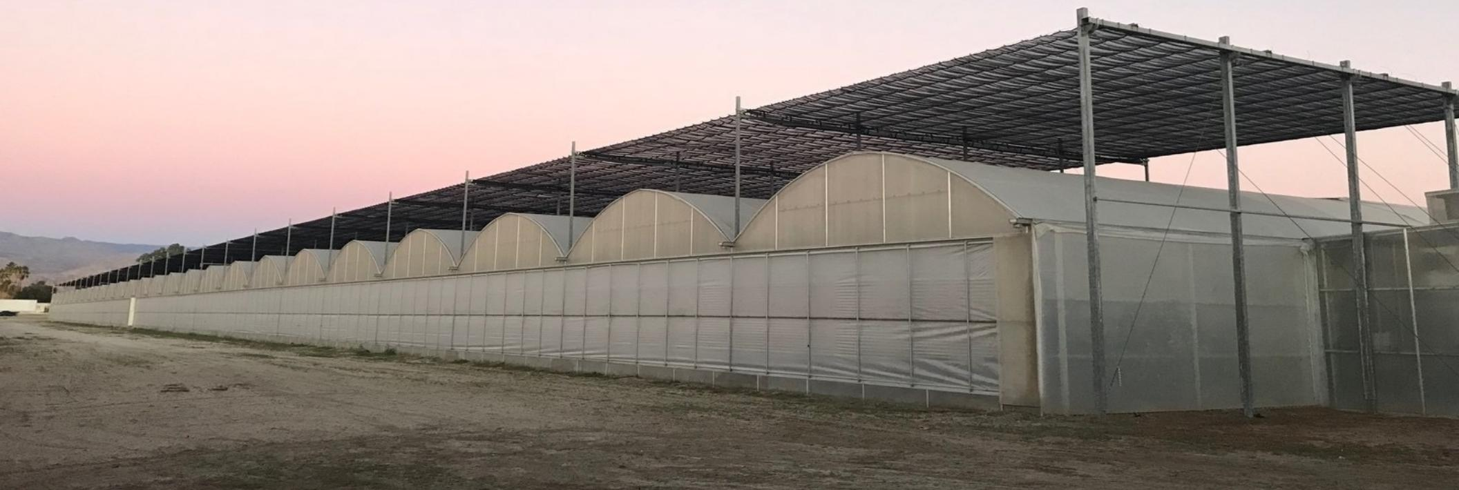
**Greenhouse #1** -249,984 SF, steel frame, automatic roof vents & computerized rollup poly side & Interior shade system, 14 Houses 24' x 744'; 12' under gutter height, constructed in 1999, 6 mil roof double poly.
