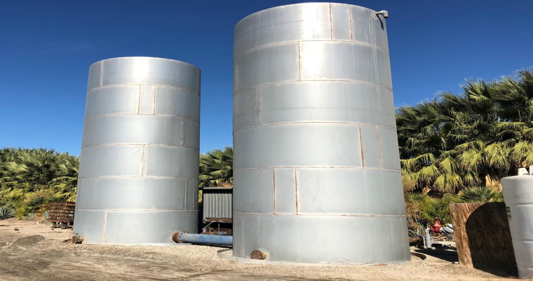
**Irrigation Well & Pumping Stations**, 800 foot deep, 500 gallons per minute, 60 HP Pump, 10" well, Twin (two) 10,000 – gallon tanks with twin 20 HP pumps for distribution to greenhouses, 2 sets of water lines (Fresh & Fertilizer) – all greenhouses plumbed, Fertilizer Injector Tank.
