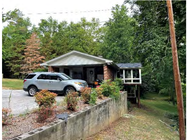
Photo 4: Eastern side of the residence, note the retaining wall.
