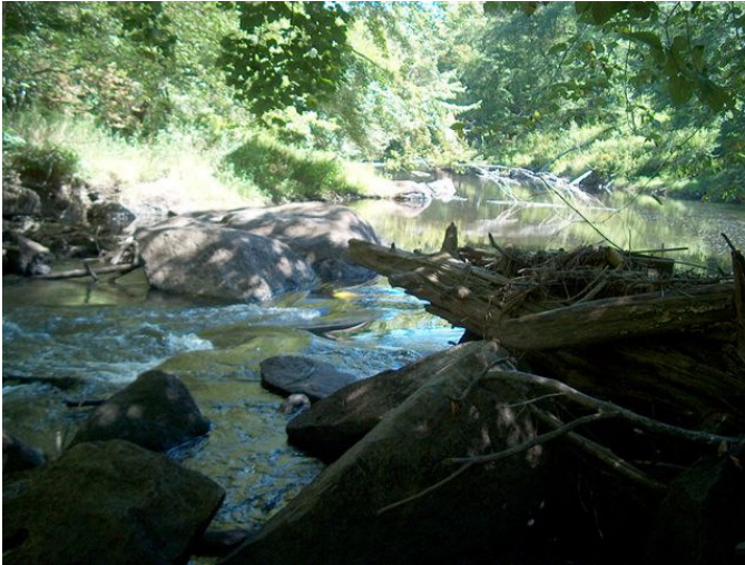
Breach on Upper Dam – 9-04-04 – Fall Flows
