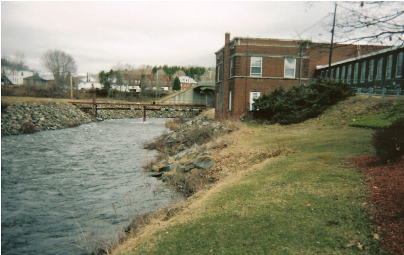
Site of Future Powerhouse beneath lower dam on east side riverbank.
