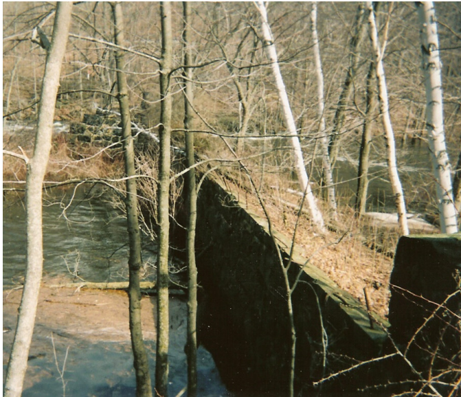
Upper Dam 4-4-05 Spring Flows.
