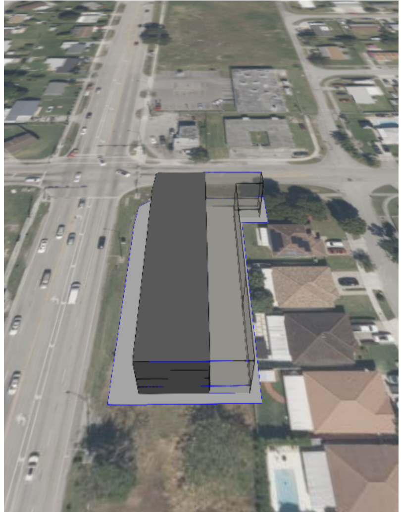
Main Building Lot Building Setback limit
