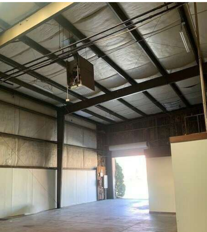
Warehouse Area w/ Drive-In Door
