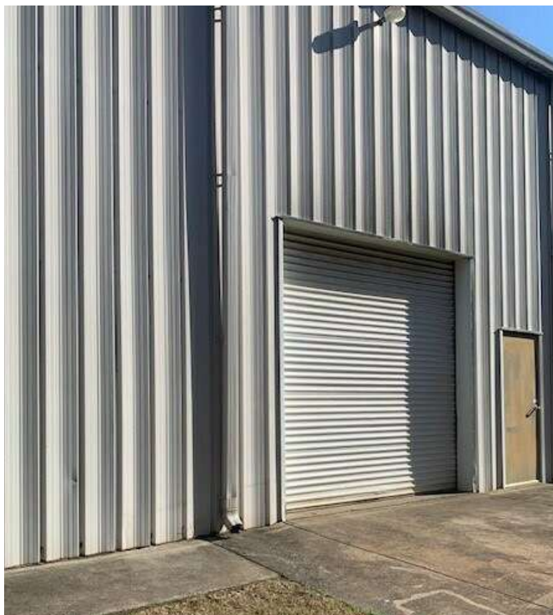
Drive-In Access. Concrete Pad to Wash Equipment
