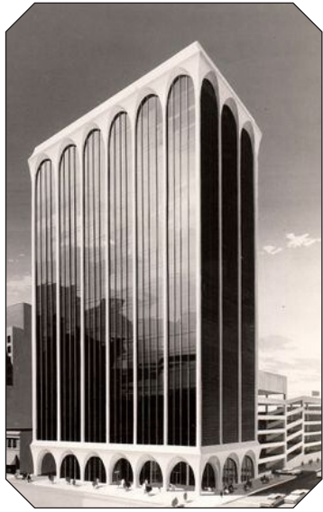
GRANT-DENEAU TOWER | 40 W. 4TH ST. DAYTON, OH 45402
