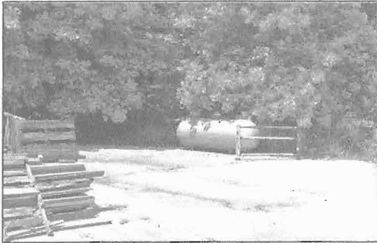
Photograph 4 Propane Tank at Rear of Building (Supplies Heat for Building)
