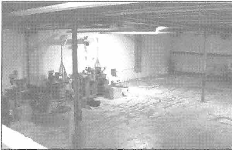
Photograph 8 Warehouse Space at Rear of Building
