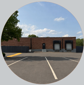
2 Loading Docks & 1 Drive-in Door
