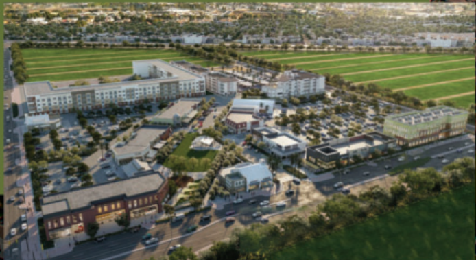
Verde Multi-Use Project (under construction)
