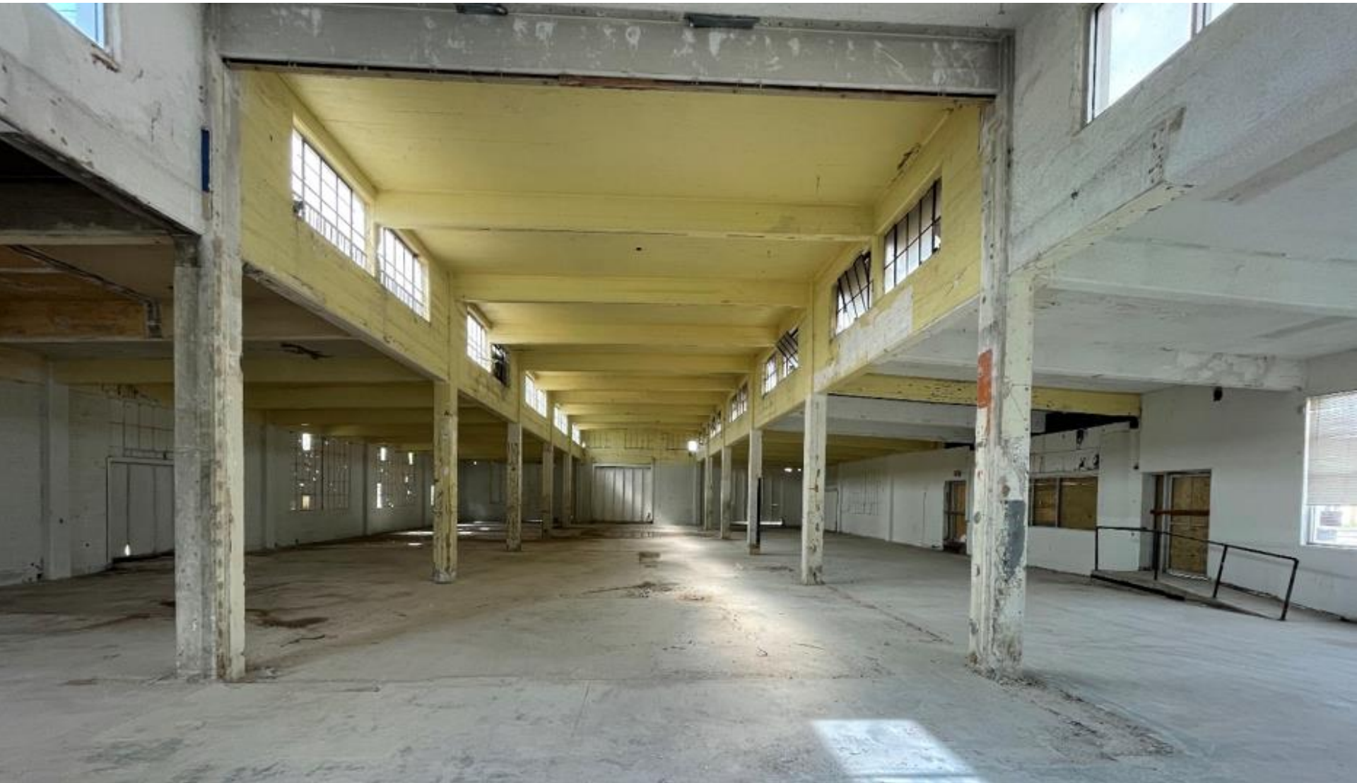
Inside the 9,100 SF building at 6614 Harrisburg
