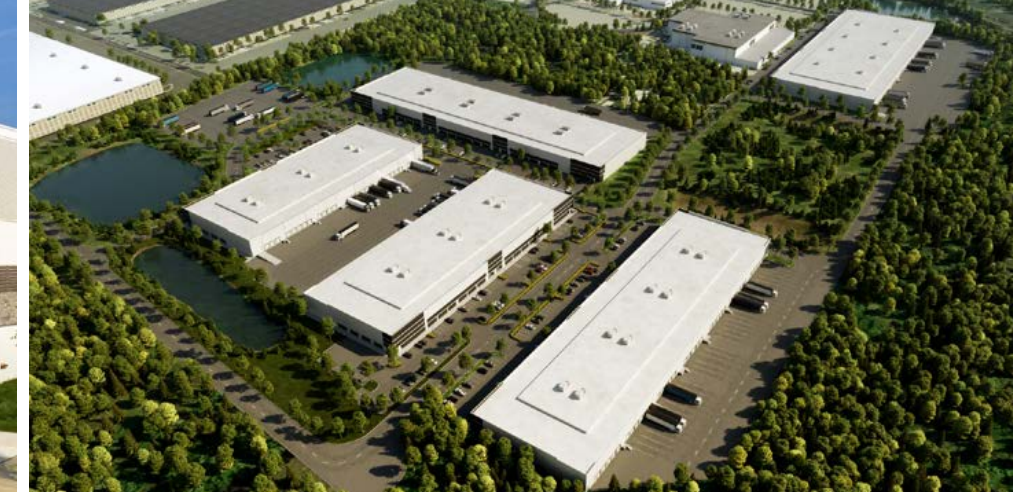
Northlake II 5-Building, 655,000 SF Industrial Park
