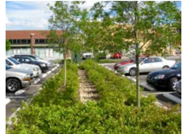
An Erie, Pennsylvania parking lot example that shows how trees, plants, and rockscaping can transform an otherwise unsightly use. The dry creek bed in the middle of this example also illustrates the functionality that can be integrated into the design for stormwater management. (Image Source: Penn State University)
