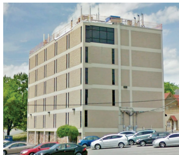
The new look of the Executive Building at 2020 W. Third St., left, reflects a more eye-catching palette than its original color scheme. The change heralds a make-over that extends throughout the interior as well. [PHOTO BY JASON BURT]
