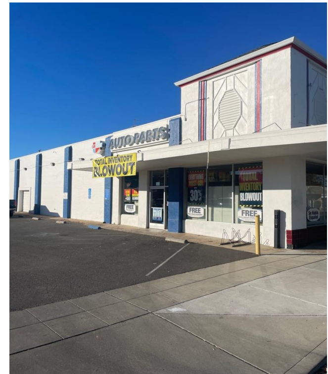
South façade looking Northwest
