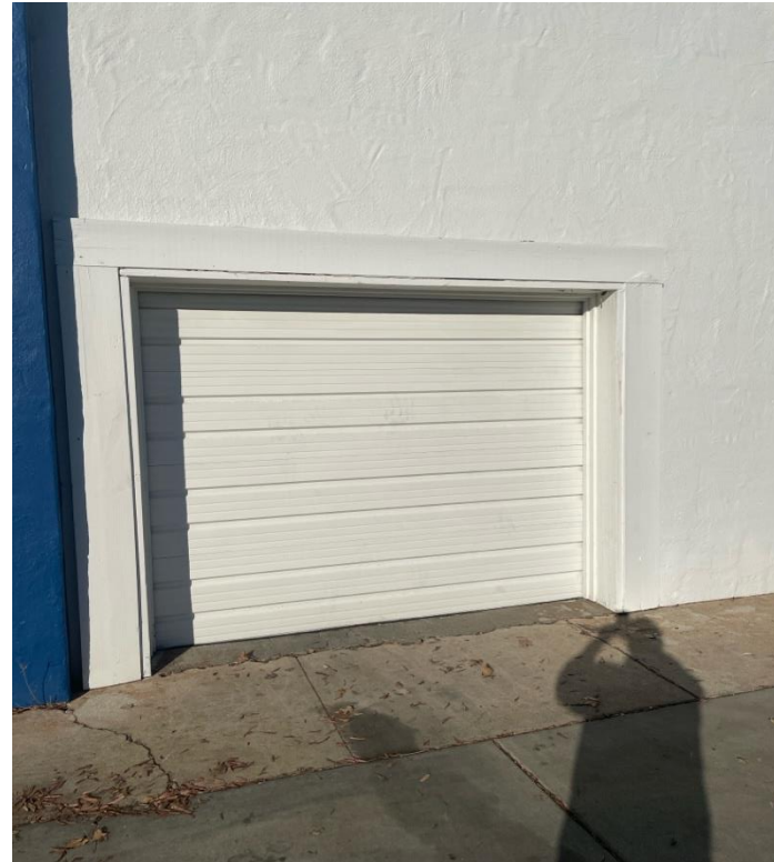
Roll- up door on Southwest side of building
