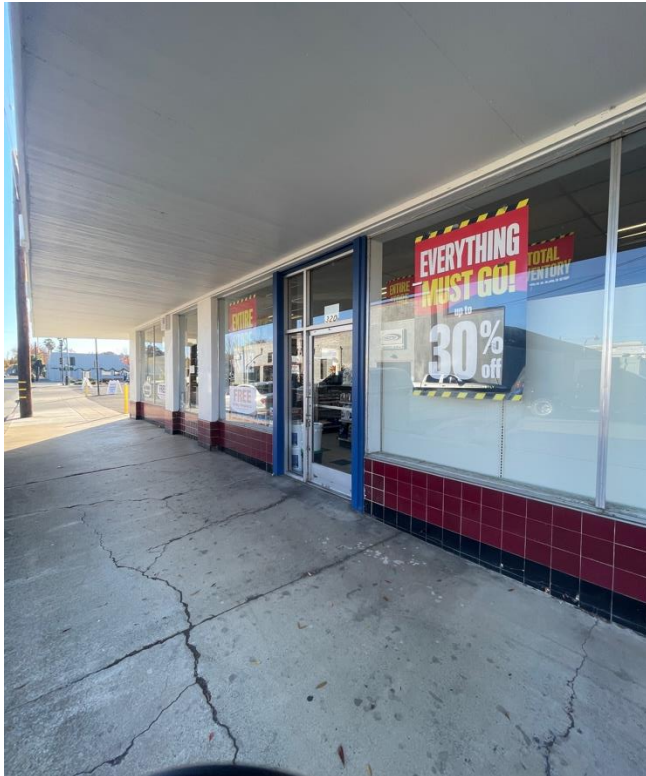
Elm Street façade looking Southwest
