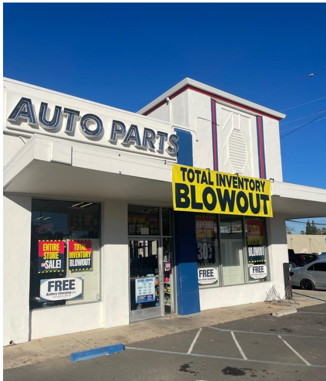
South façade looking North
