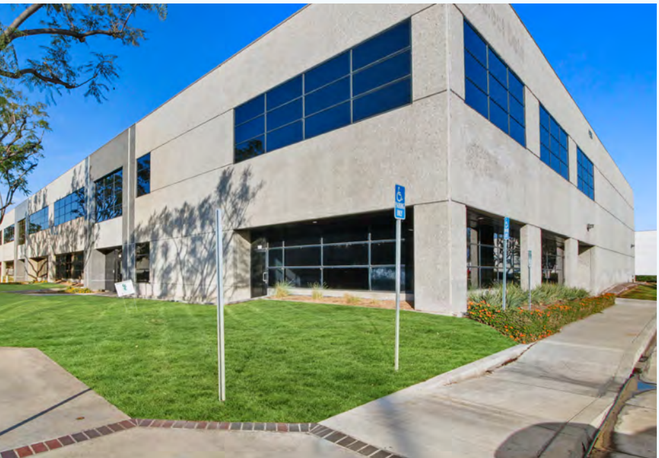
*Second Floor Office
