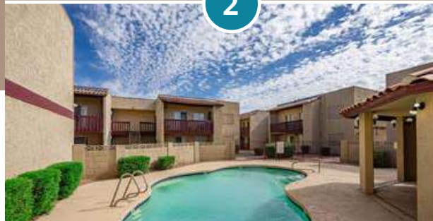
CORONA DEL SOL 27 EAST CORONA AVENUE | PHOENIX
