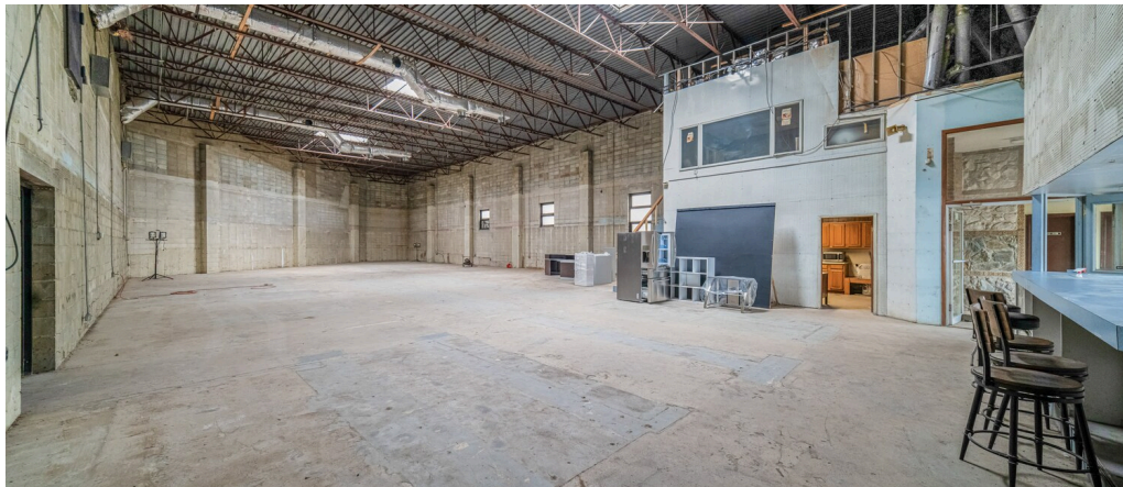
Main warehouse — high bay open-span layout with skylights and steel trusses
