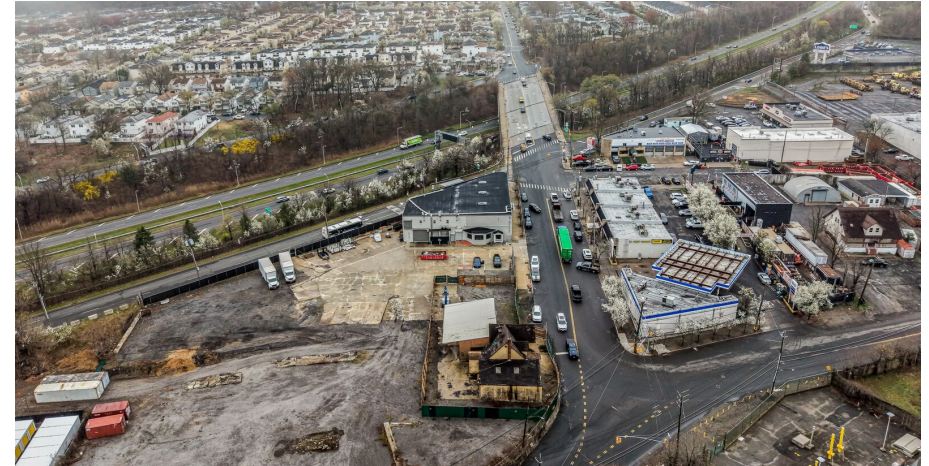
Aerial context — full lot extent, street-to-street configuration, and Route 440 access
