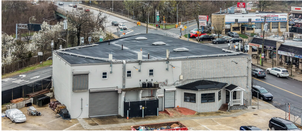
Close aerial — building at Bloomingdale Road / Veterans Road with Route 440
