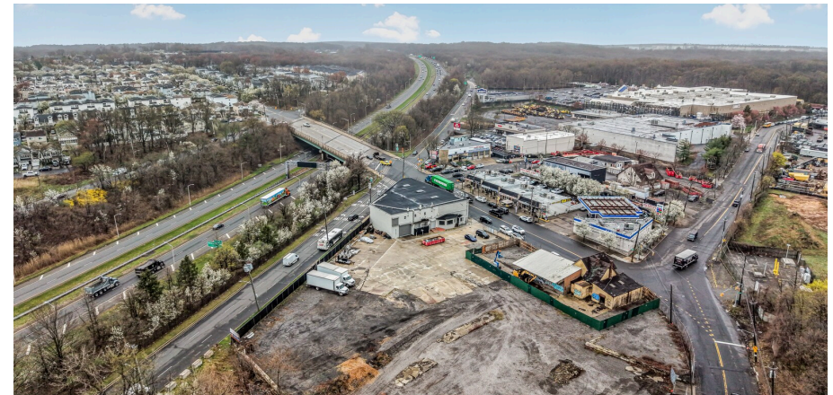
Wide aerial context — Route 440 corridor and surrounding West Shore commercial market
