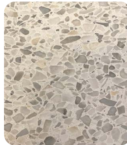
TERRAZZO FLOORING AT LOBBY
