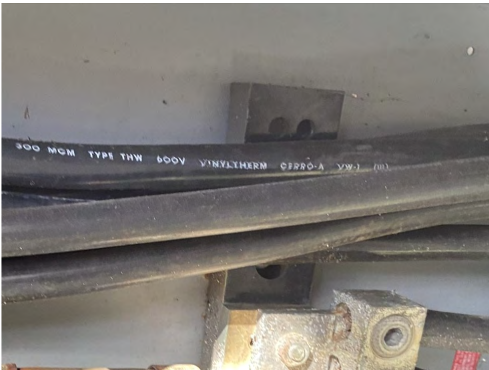
13. View of Wires and Cables
