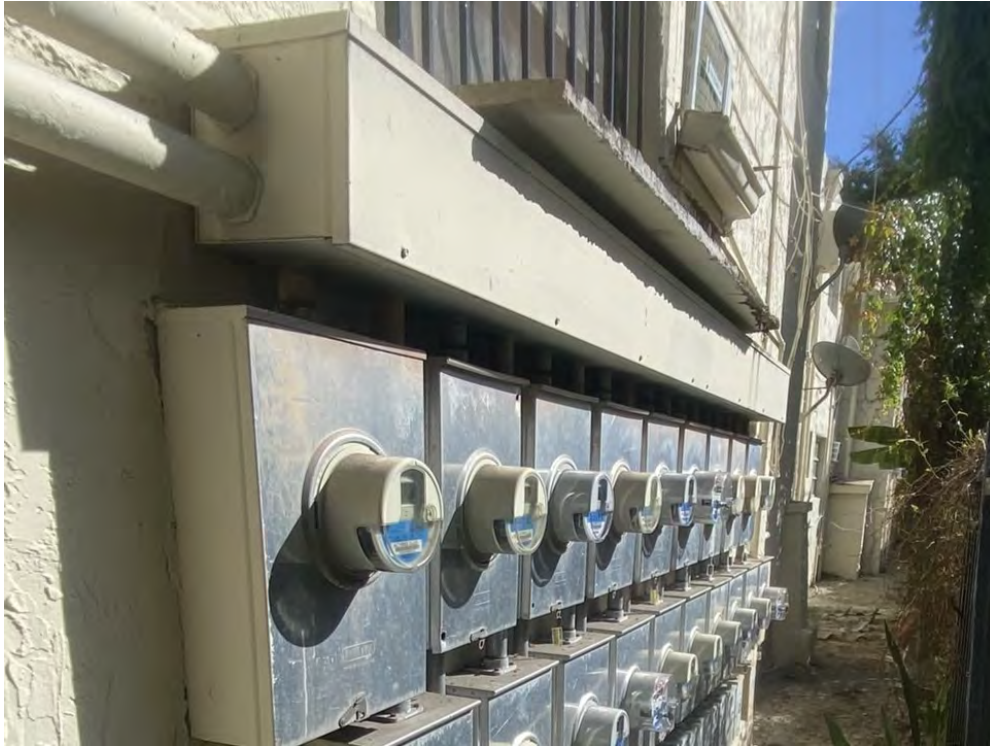
6. View of Electrical Gutters, Wireways
