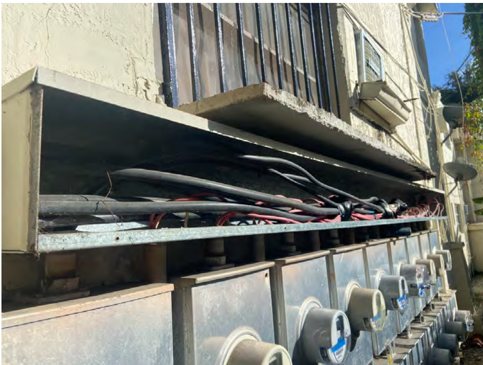
6. View of Electrical Gutters, Wireways
