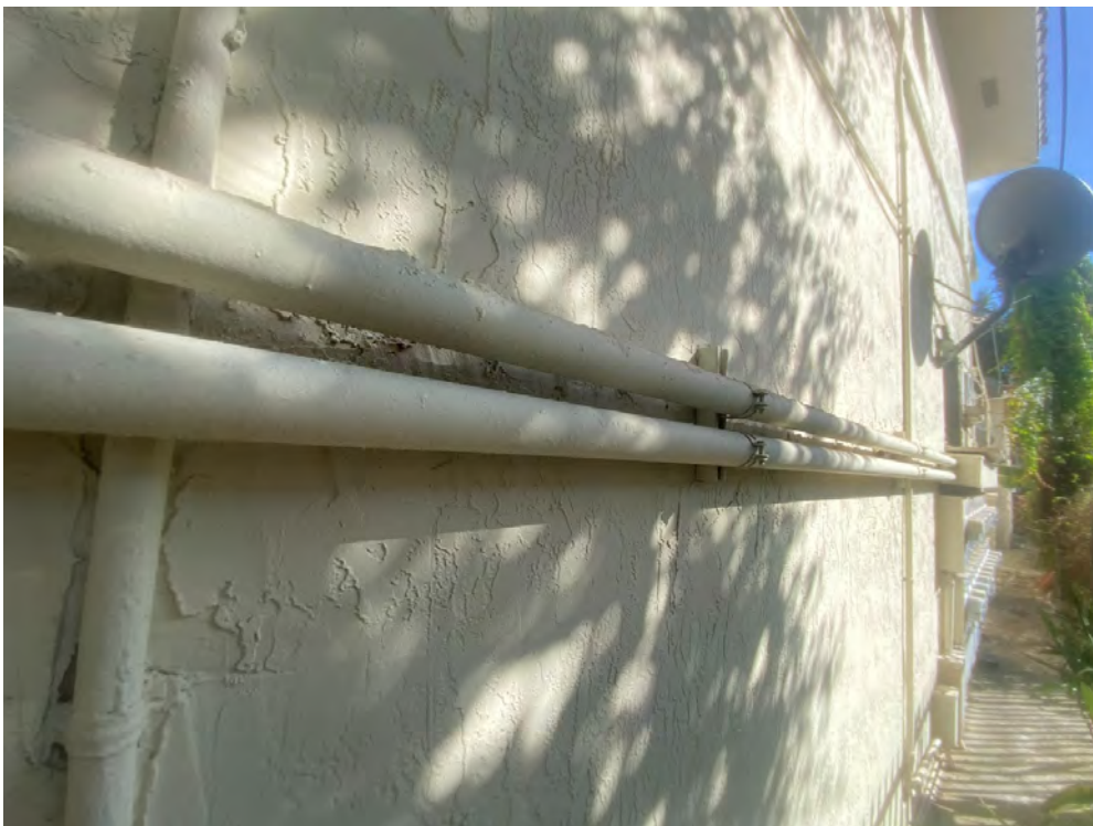
11. View of Service Conduit/Raceways
