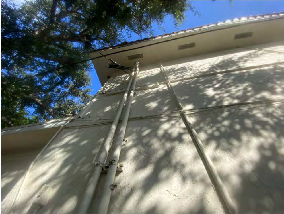
11. View of Service Conduit/Raceways
