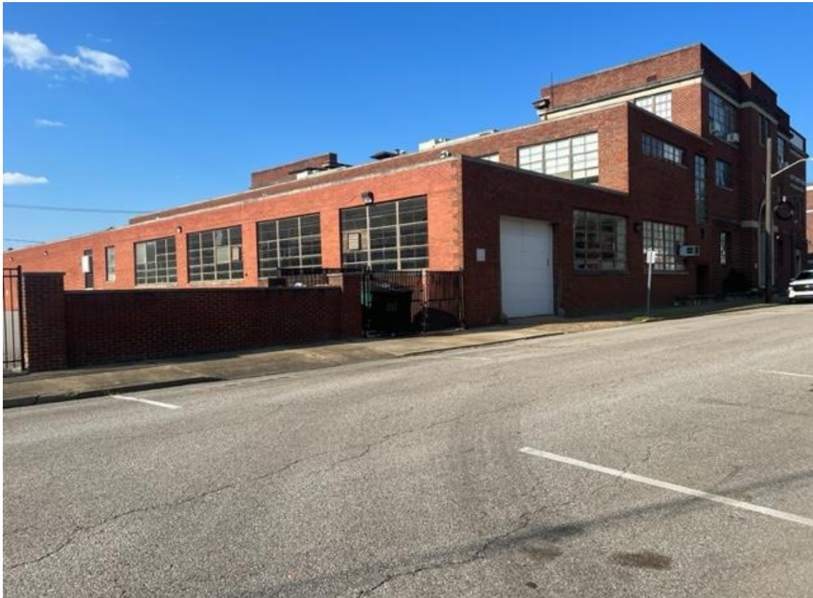
Shrewsbury Street frontage. Mezzanine is the two story space shown.
