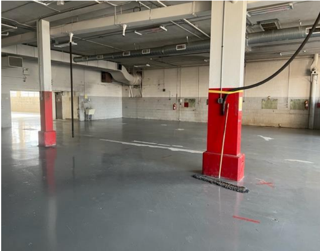
Separating wall between portions
