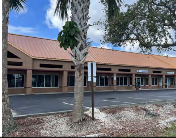
Front Left Side of Building
