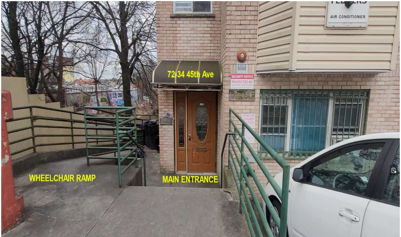
FRONT MAIN ENTRANCE (Note wheelchair ramp)
