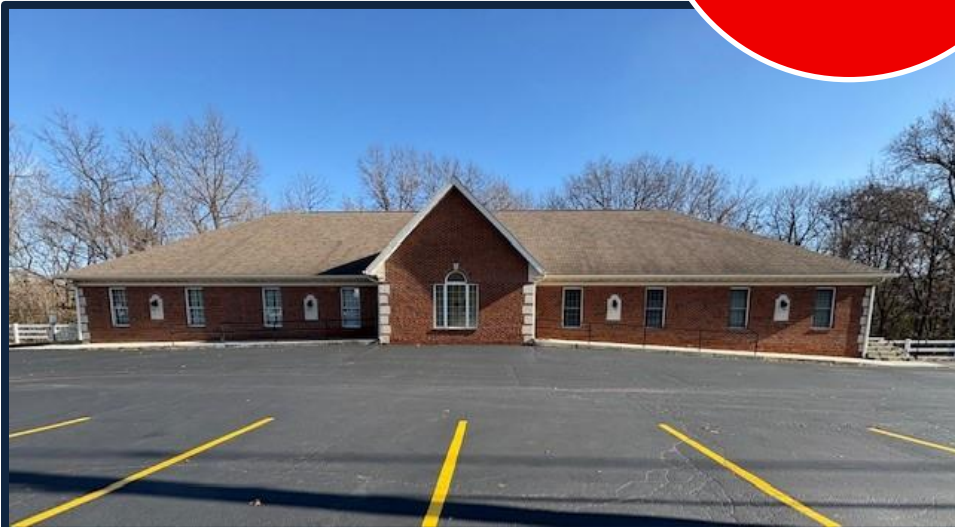
9,600 SF PROFESSIONAL OFFICE BUILDING
