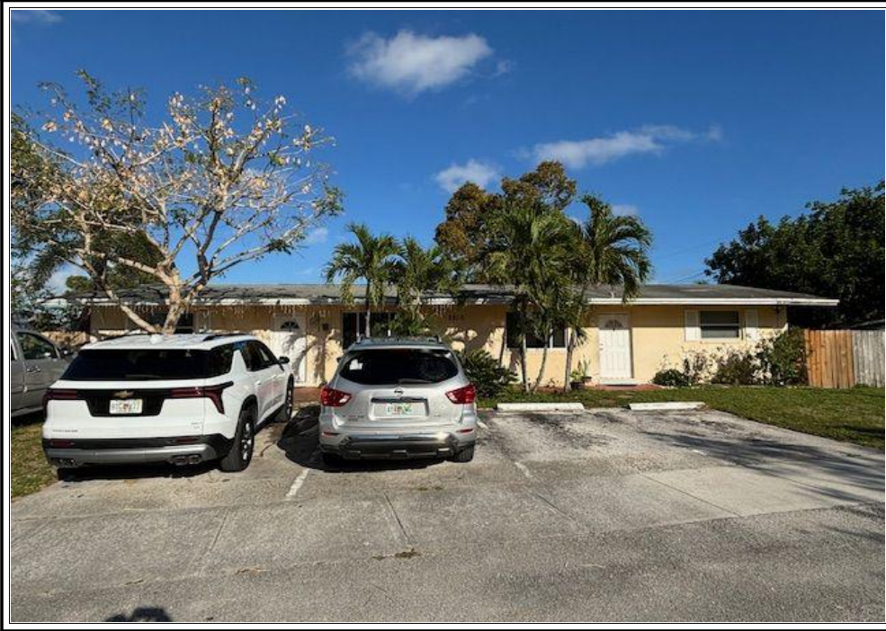
FRONT OF SUBJECT PROPERTY 2200 SW 42nd Ave Fort Lauderdale, FL 33317
