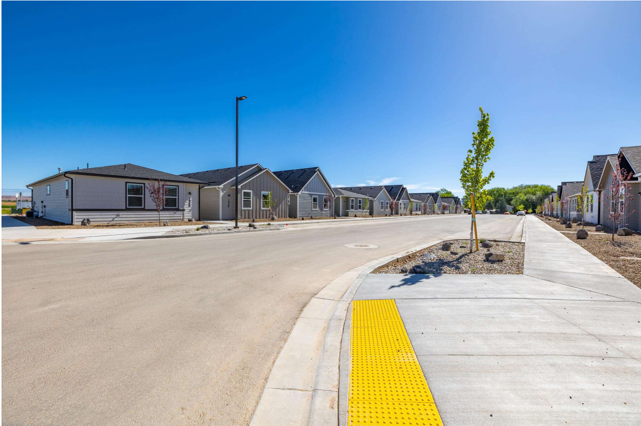
Street view of the Turner House Depot community
