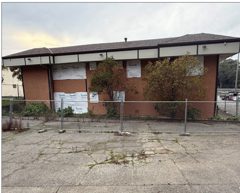
Current Exterior Condition
