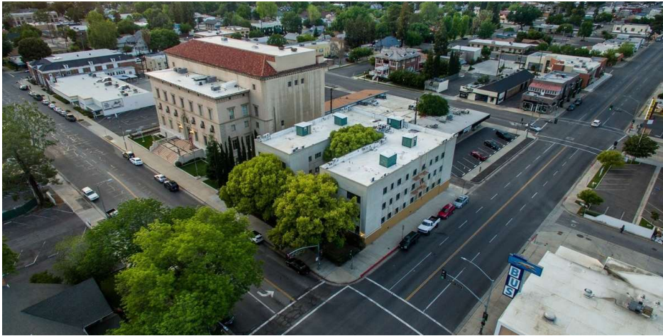
★ The New Yorker Apartments 1906 18th St, Bakersfield, CA 93301
