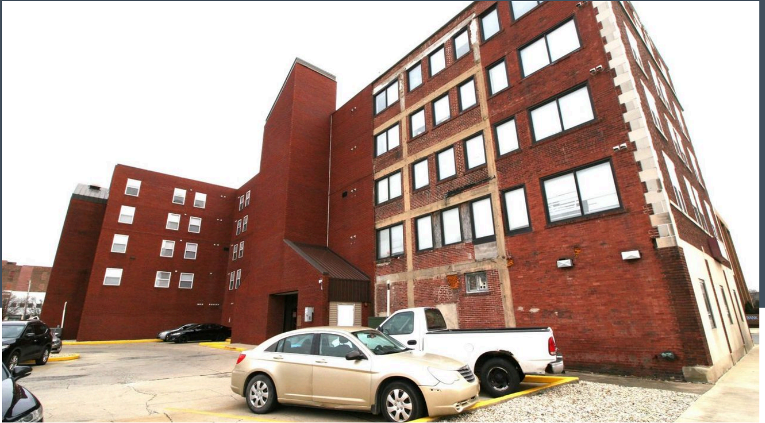
Rear Parking Lot
