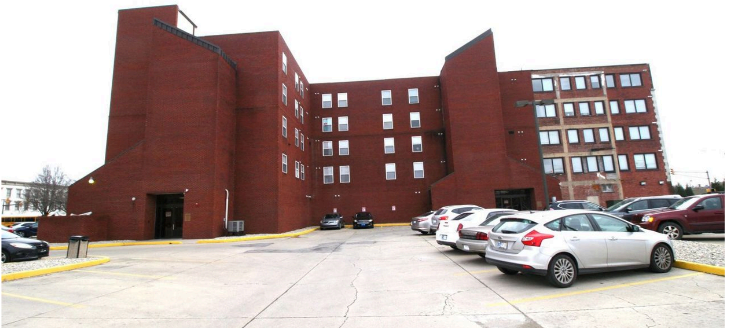
Rear Parking Lot
