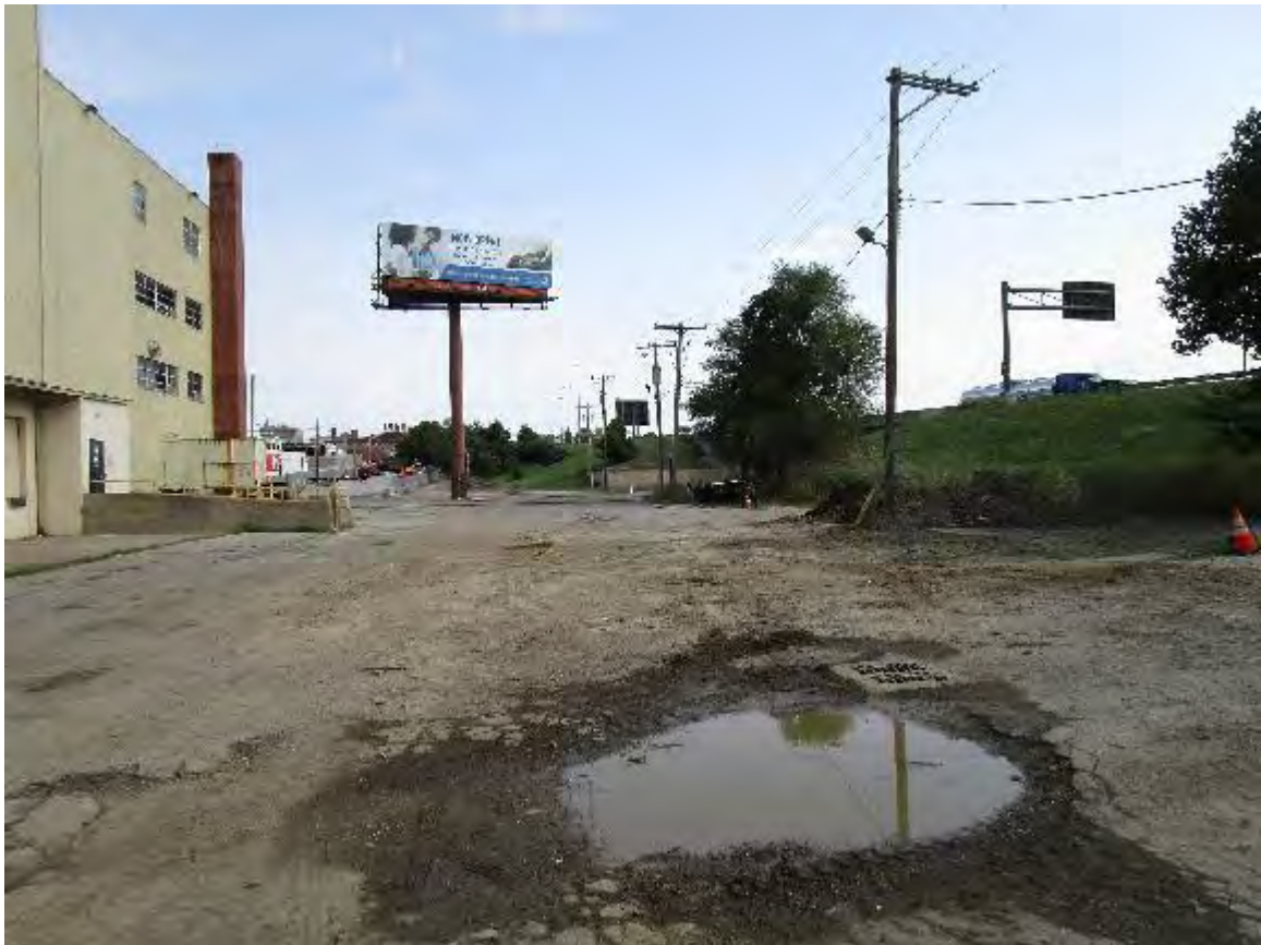
East parking lot
