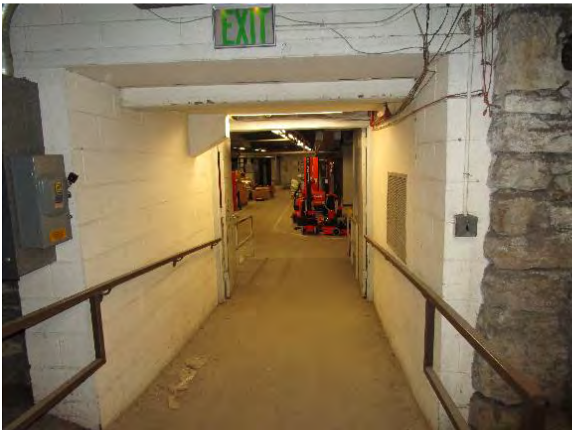
Basement-showing old basement to new basement
