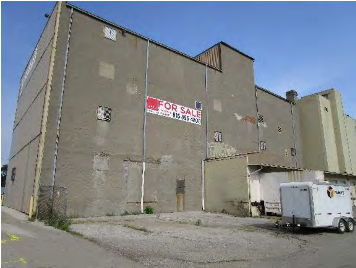
East side of building
