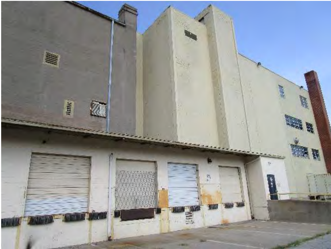
East side of building
