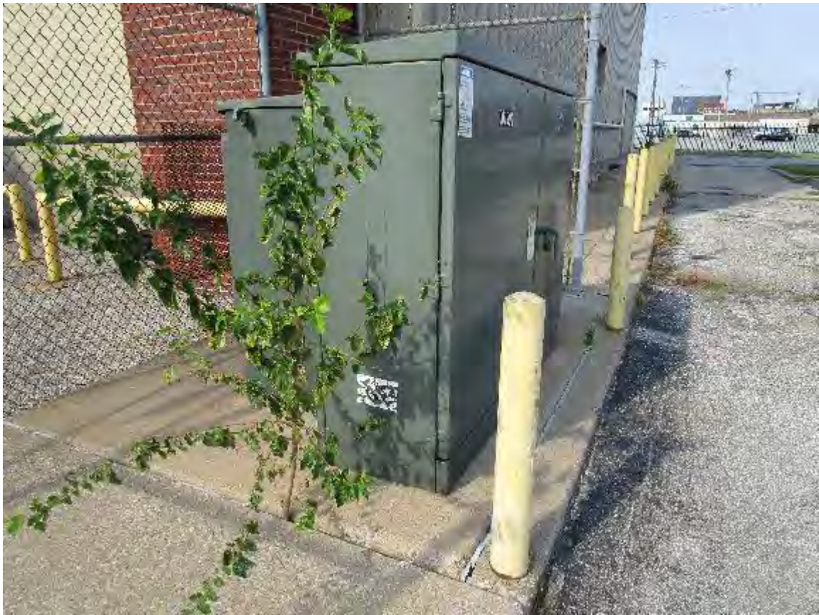
Pad-mounted transformer
