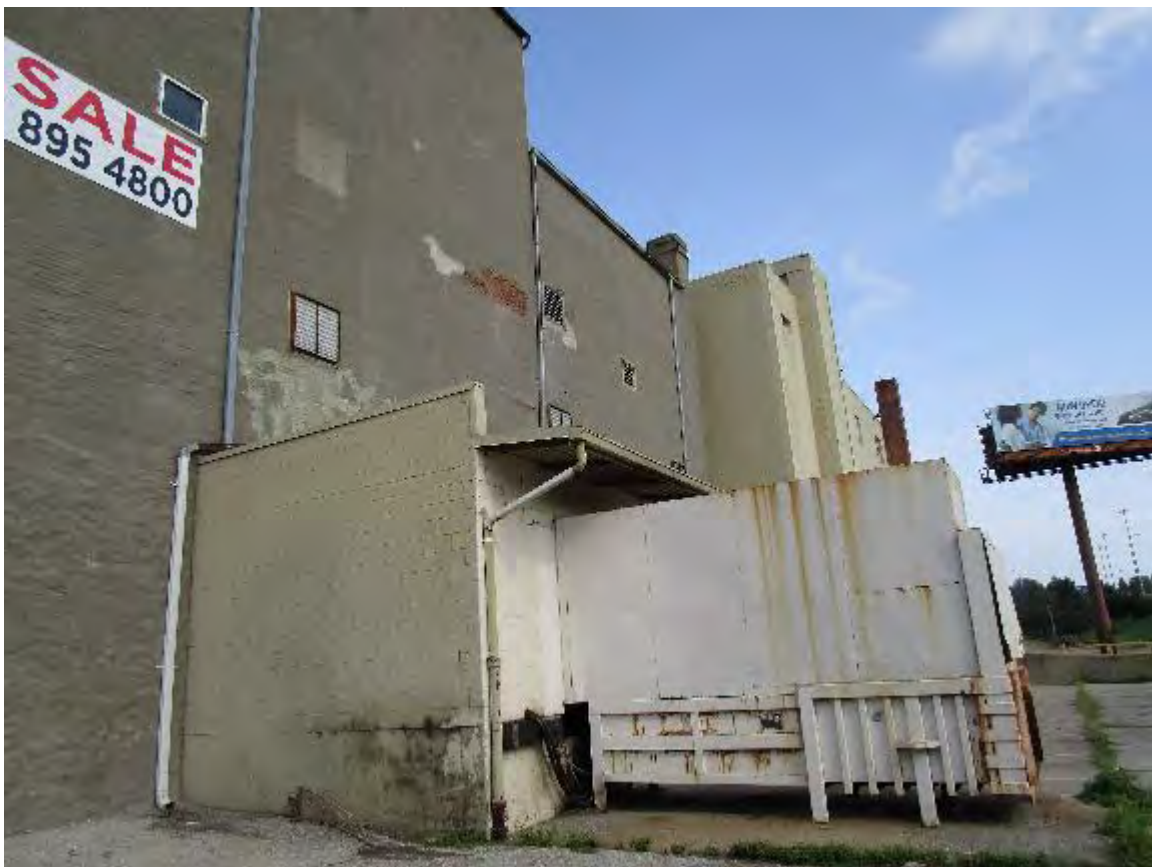
East side of building
