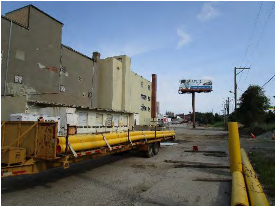
East parking lot
