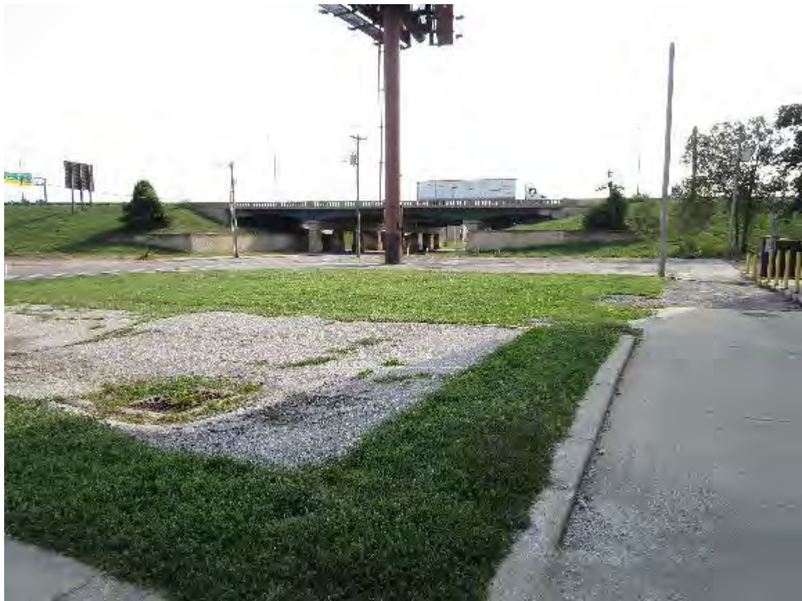
North portion of subject property
