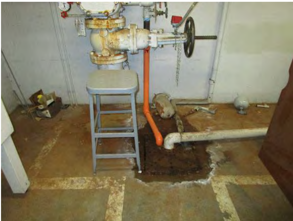
New basement showing floor drain
