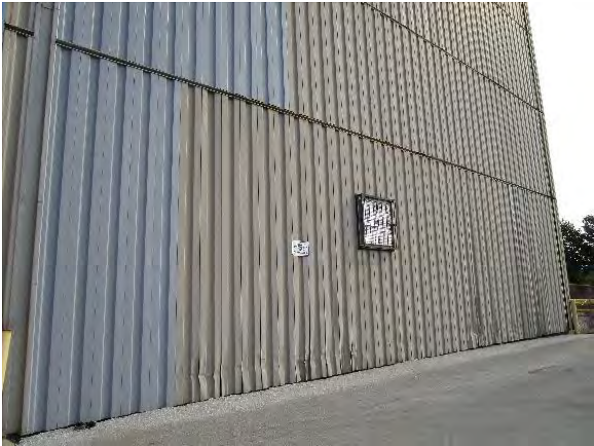
South side of building
