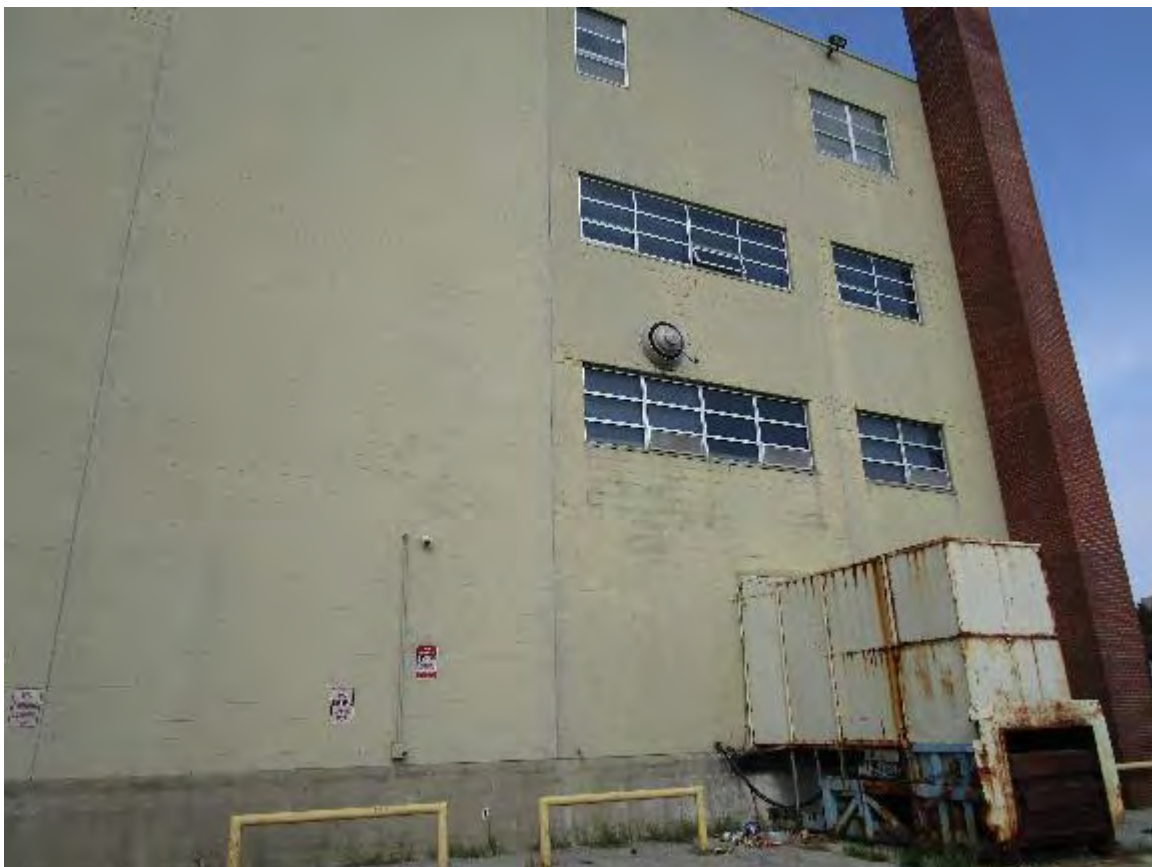
East side of building
