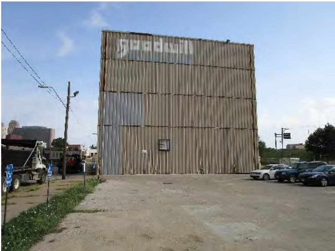
South side of building/property
