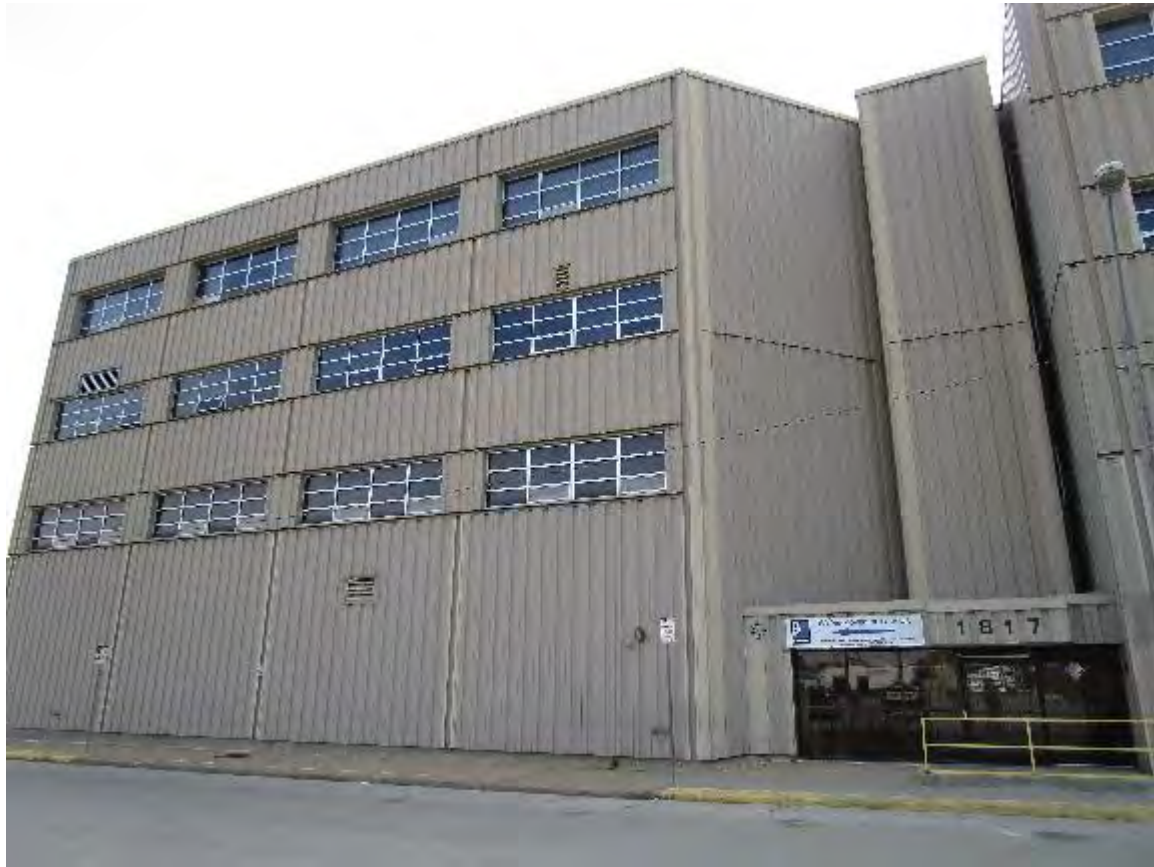
West side of 1970s addition
