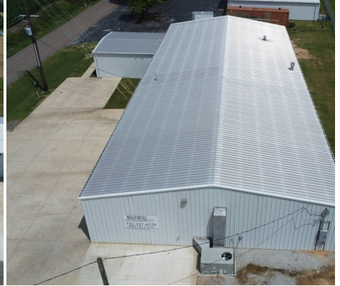
OVERHEAD • ROOF &amp; LOT
