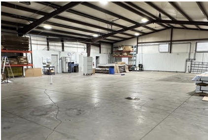
OPEN CLEAR-SPAN BAY
