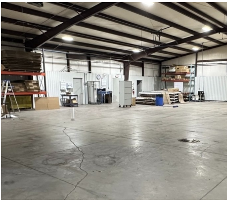
OPEN CLEAR-SPAN BAY
