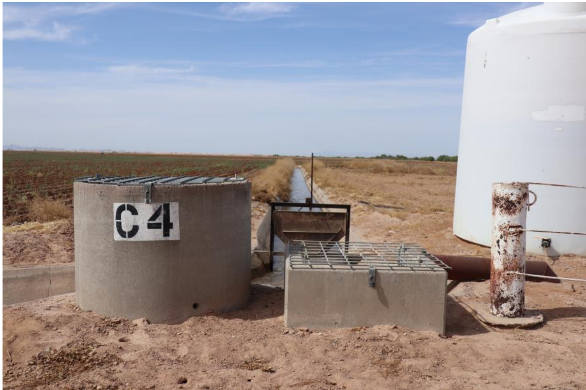
CAIDD irrigation water delivery turnout
