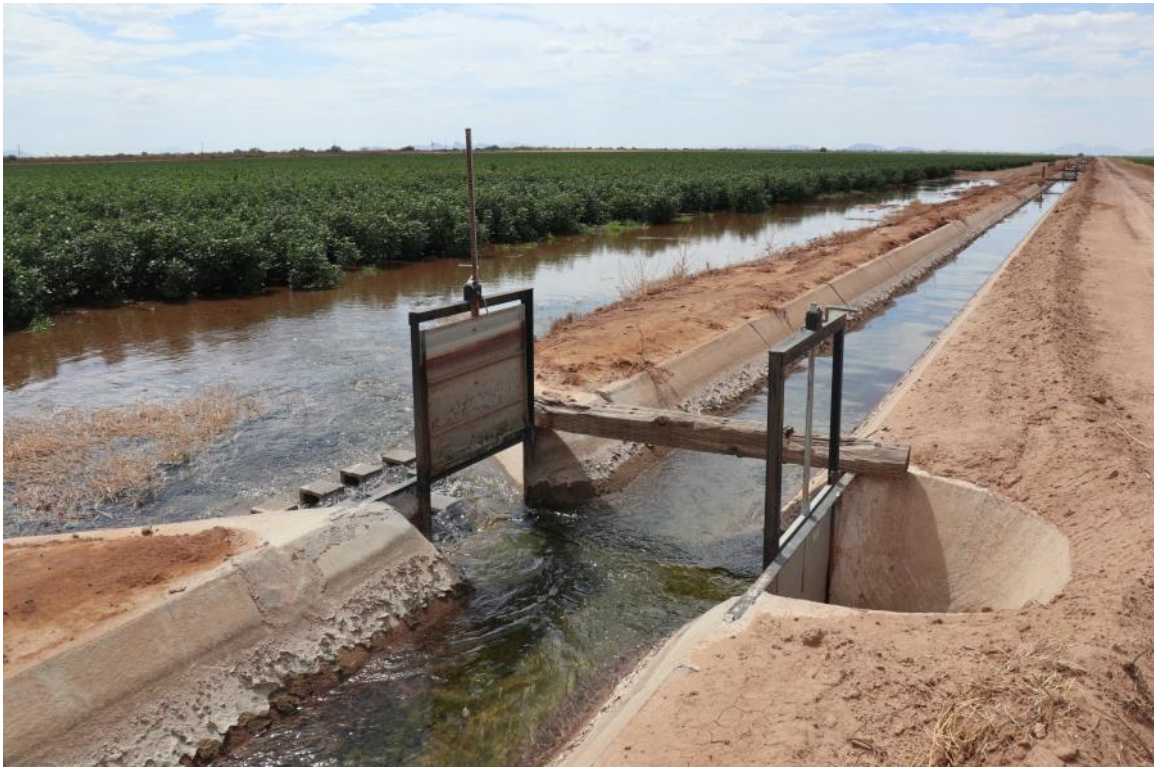
Concrete ditch with irrigation water turnout
