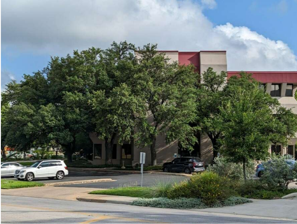
Front of Building
