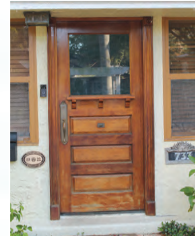
This three-panel door with a single large light resting on a sill is a common Wood Frame Vernacular door
