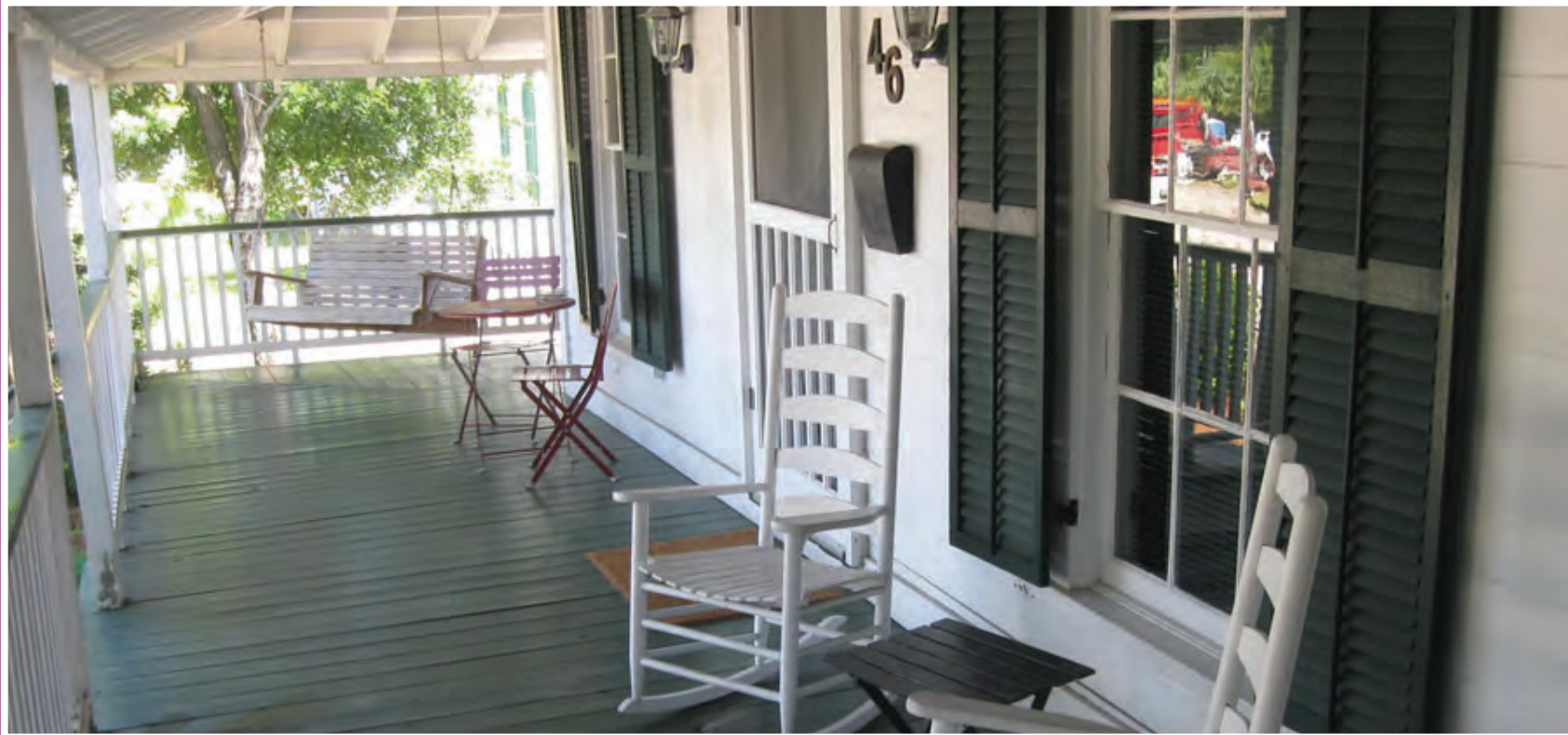
Wrap-around porch in an Apalachicola, Florida home.
