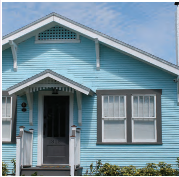
Four over one wood double-hung windows grouped in pairs
