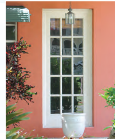
This 15-lite "French" door is also a common door type in the Wood Frame Vernacular style
