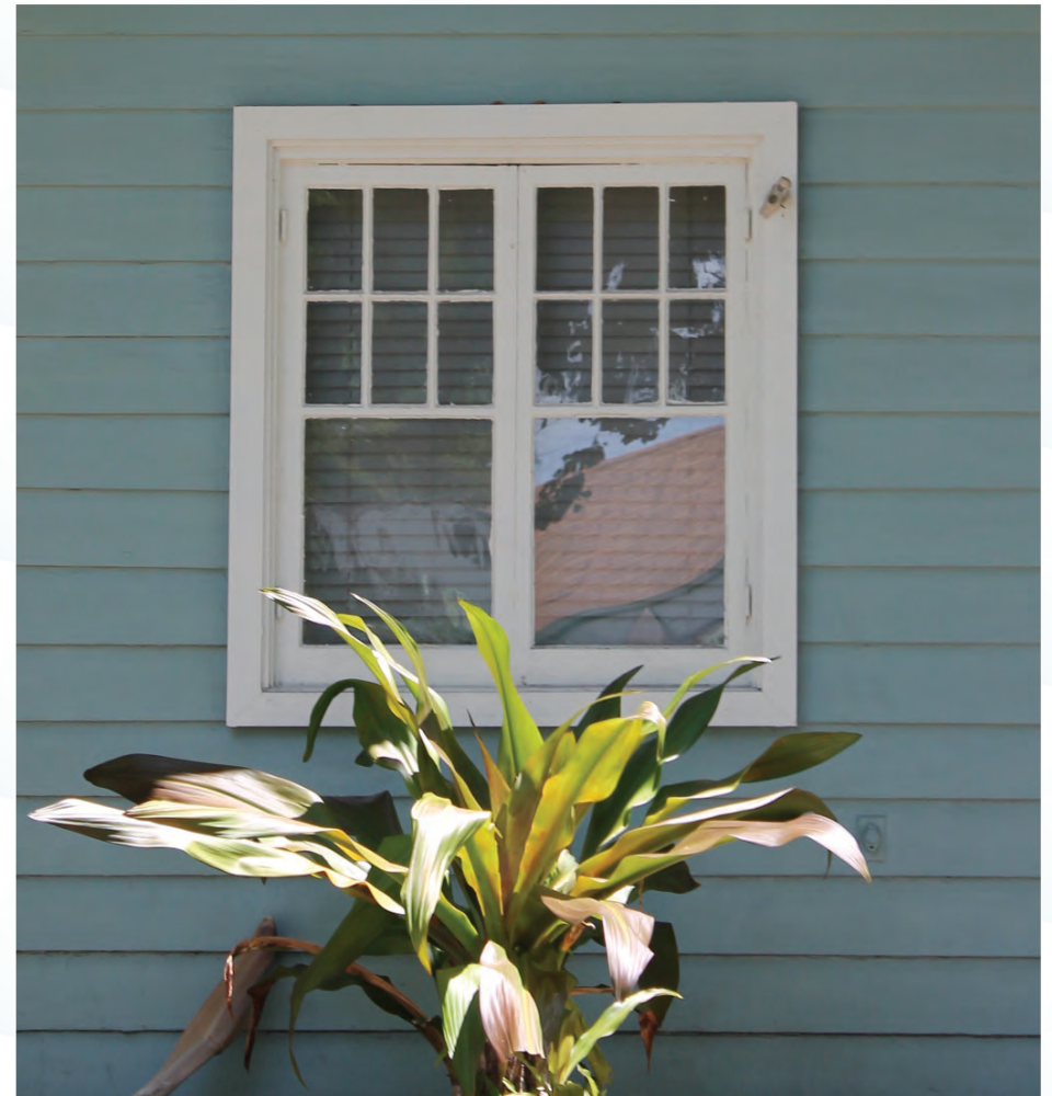
These are paired six over one wood casement windows
