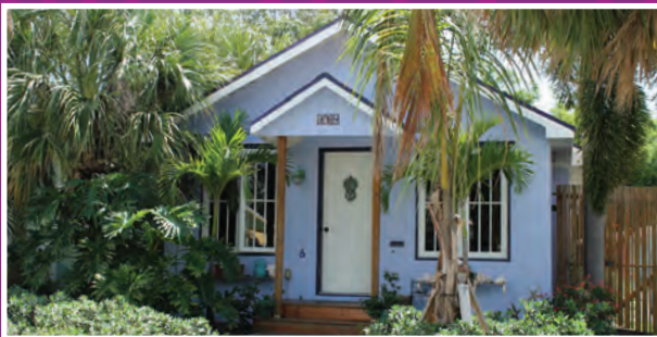
Paired three over three windows
