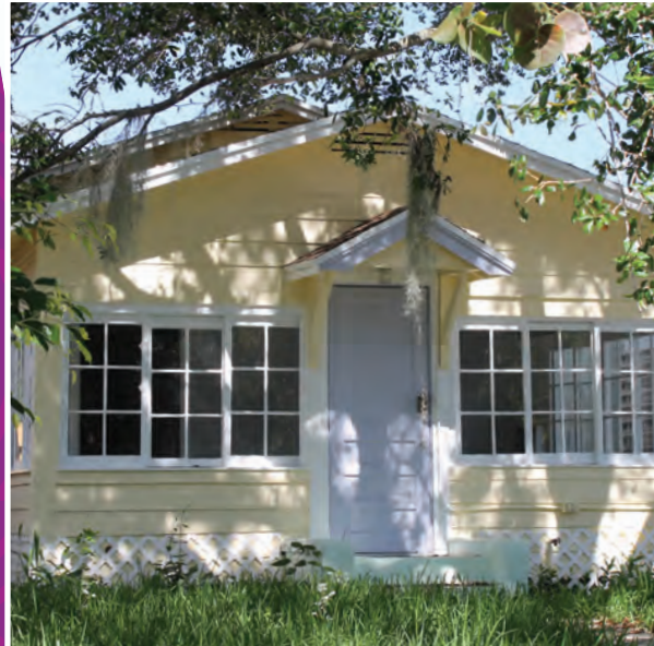
Multi-light wood casement windows in a Wood Frame Vernacular porch
