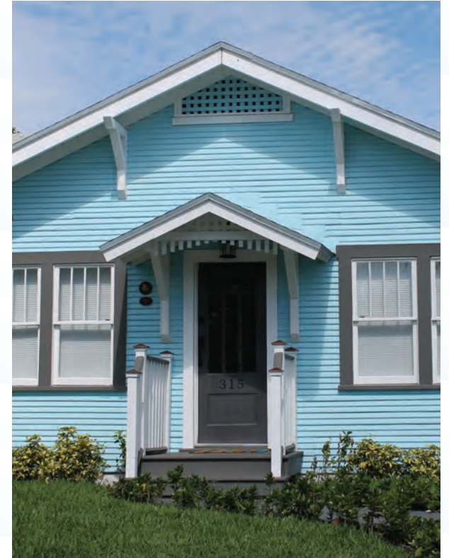
Wood Frame Vernacular house with gable end stoop overhang, Lake Worth Beach, Fla.
