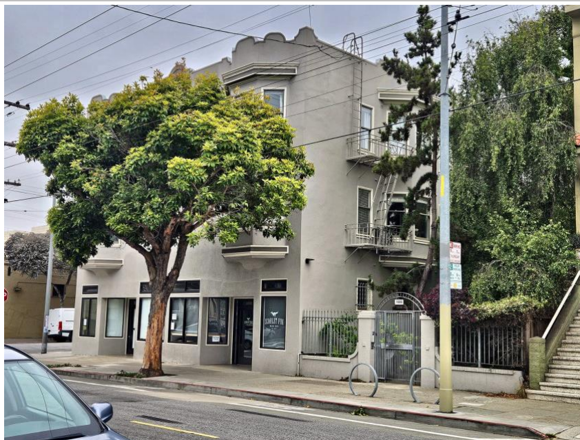
1686 Hayes Street — corner mixed-use frontage with ground-floor wine bar and gated residential entry
