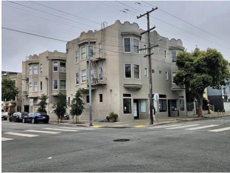
Corner elevation — bay windows & fire escapes
