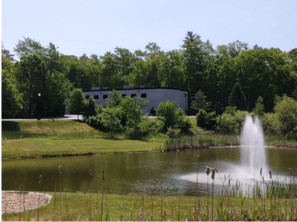
Rear of facility
