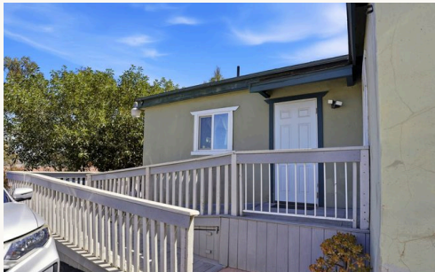
EXTERIOR – ACCESSIBLE ENTRY
