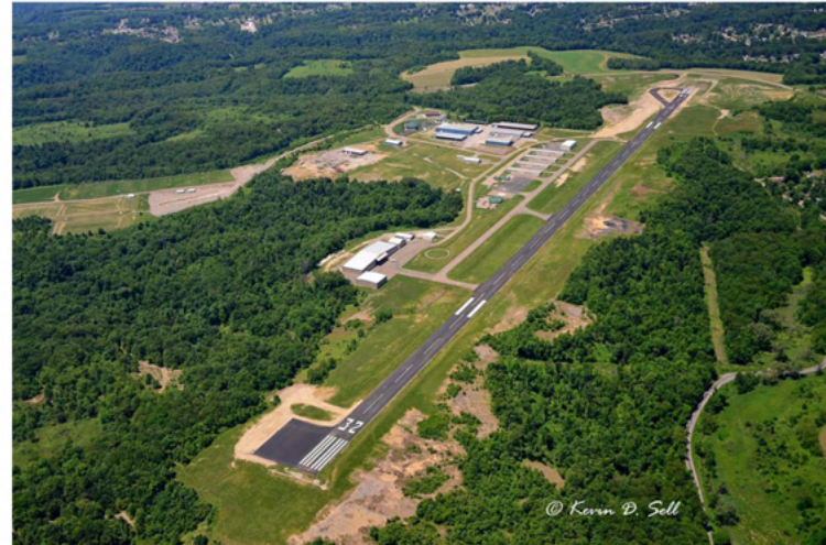
The Runway 14-32 Extension project, completed in 2014, provides the capability to serve the needs of the corporate tenants and transient users of Jefferson County Airpark.
