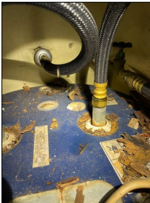
53. Equipment leaking
