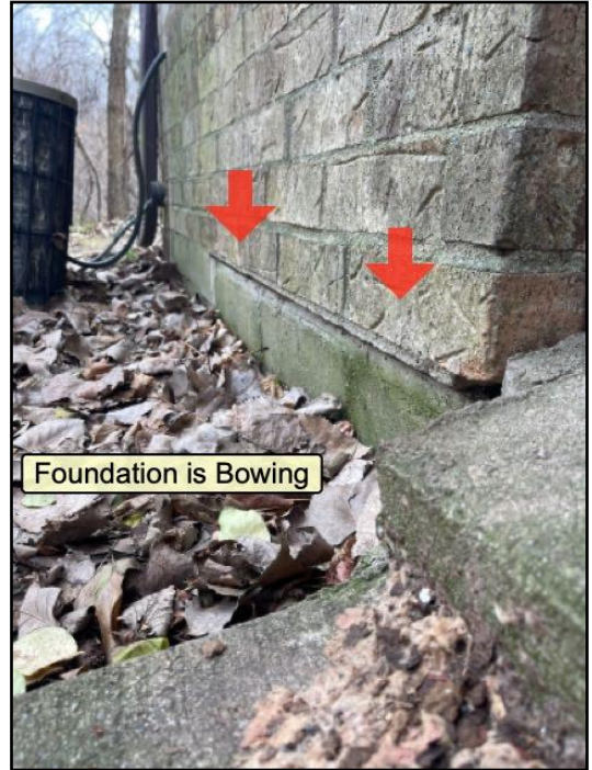
93. Cracked - settlement
