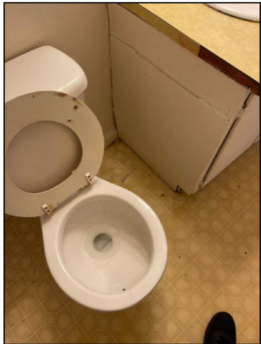
50. The overall condition of the structure was...
