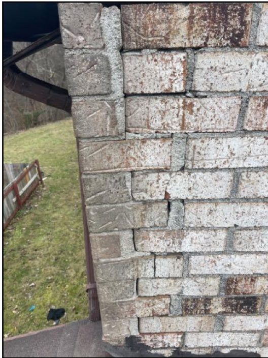
103. Mortar deterioration
