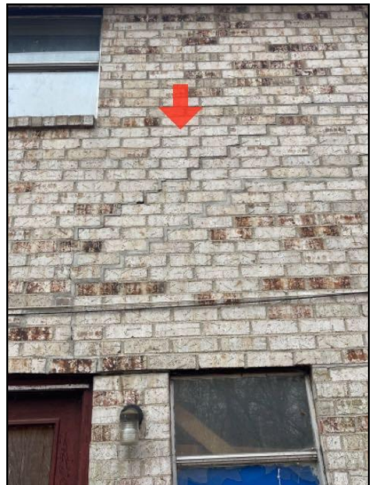
95. Cracked - settlement
