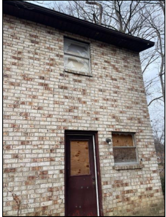
108. Cracked - settlement
