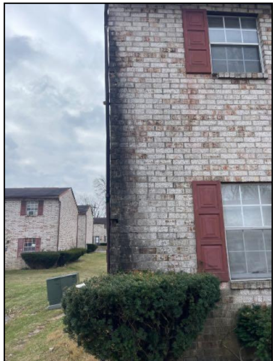
106. Mortar deterioration
