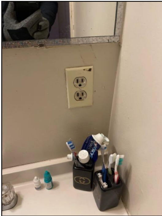
27. The Installation of ground fault circuit...
