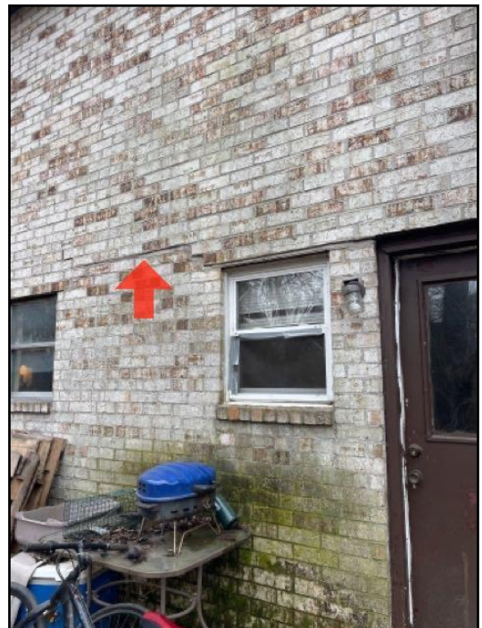
99. Cracked - settlement
