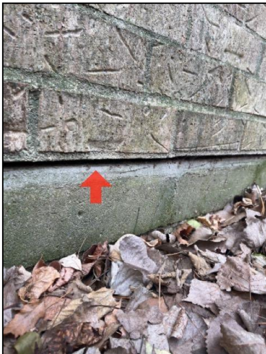
94. Cracked - settlement
