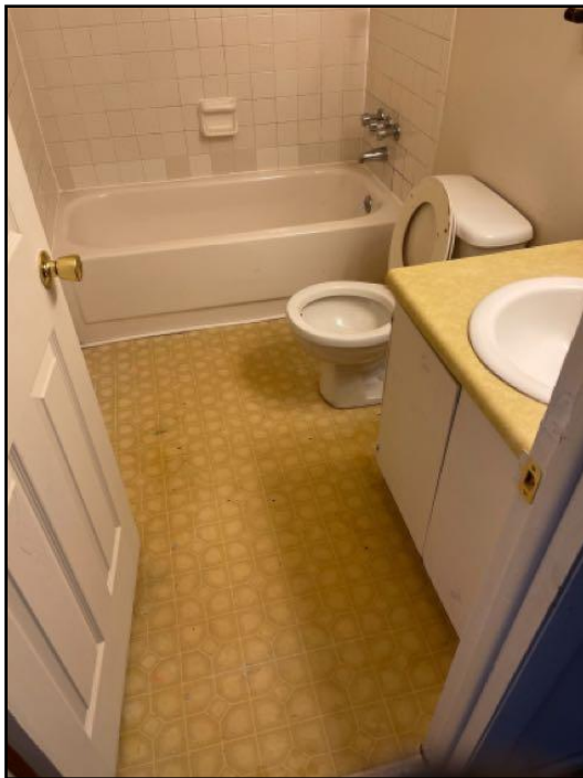
49. The overall condition of the structure was...
