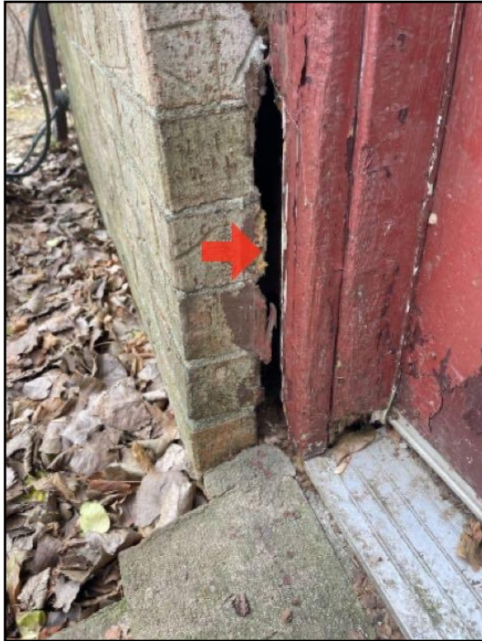
92. Cracked - settlement
