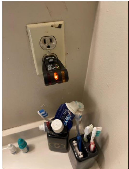
28. The Installation of ground fault circuit...
