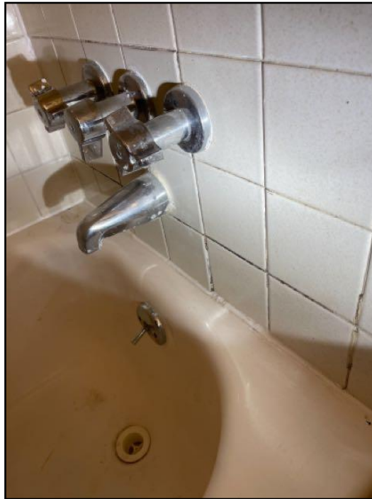
51. The overall condition of the structure was...
