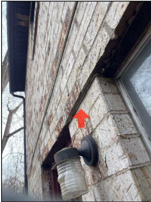
96. Cracked - settlement
