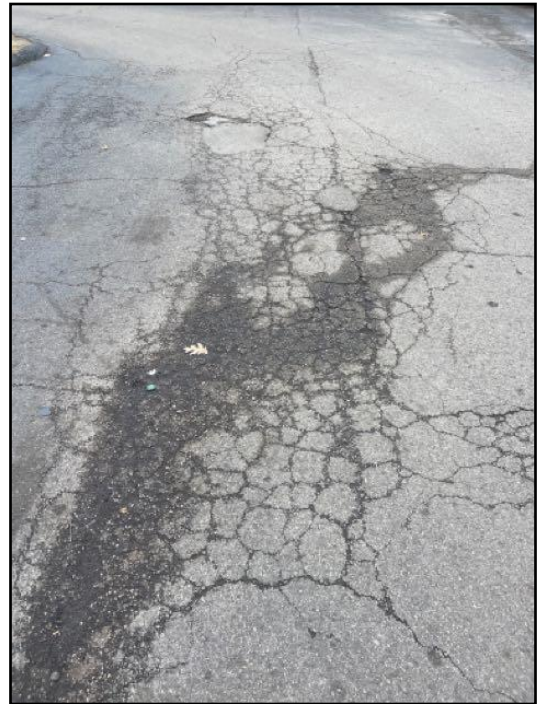
149. Cracking
