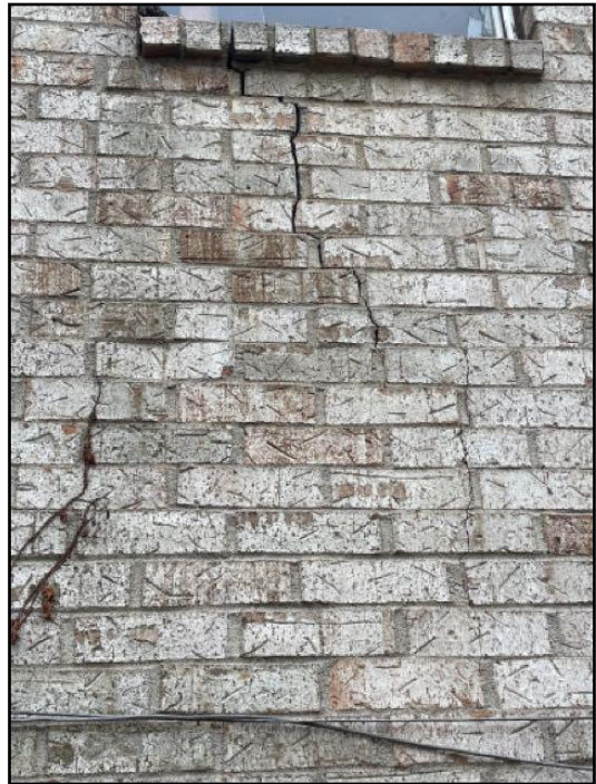
104. Mortar deterioration
