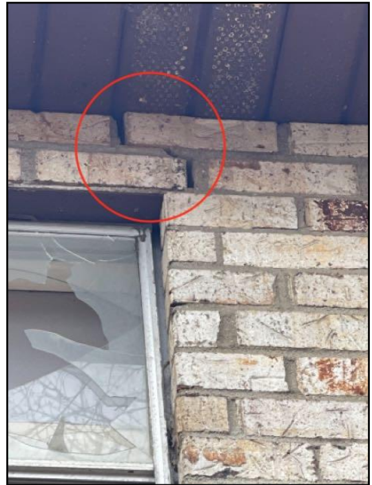
97. Cracked - settlement
