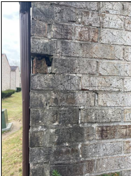
105. Mortar deterioration
