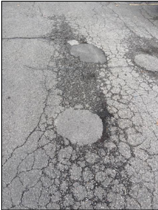
148. Cracking
