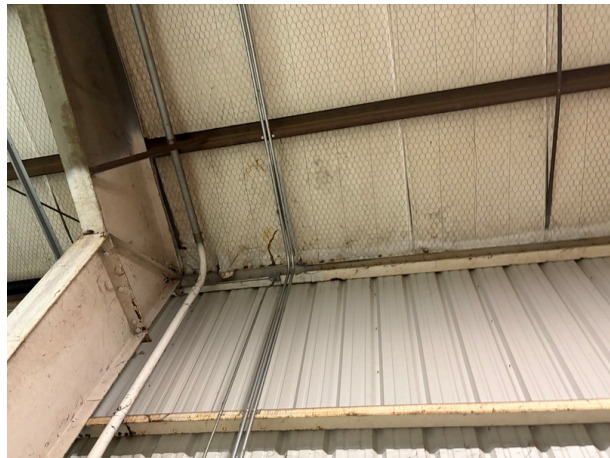
View of roof by southern portion of the building
