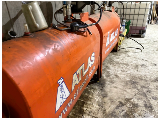
ASTs with some staining observed and a tote in the background.
