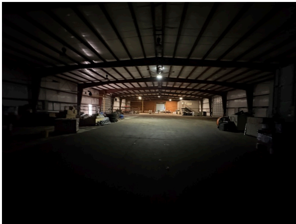
View of northern portion of the building
