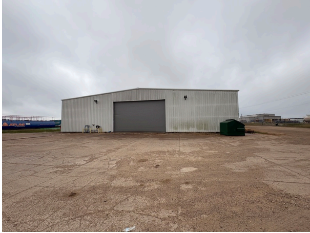
View of southern exterior of the building
