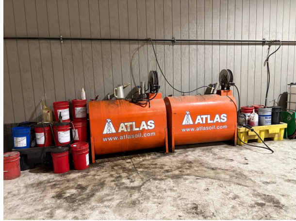
ASTs and 5 gallon buckets stored on concrete with staining observed in the vicinity. Additional 5 gallon drums on the right stored on a spill pallet.
