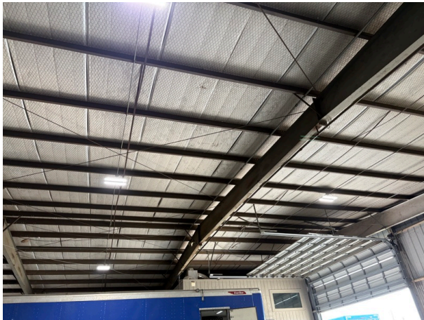
Roof in the southern portion of the building
