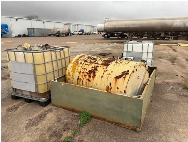
An AST in secondary containment and two IBC totes.
