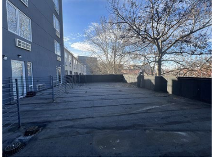
SECOND FLOOR TERRACE
