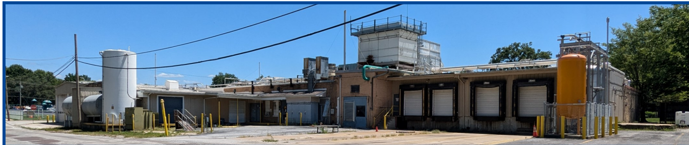
Back of Building facing W. 5th Street
