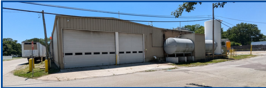
Back of Building facing W. 5th Street
