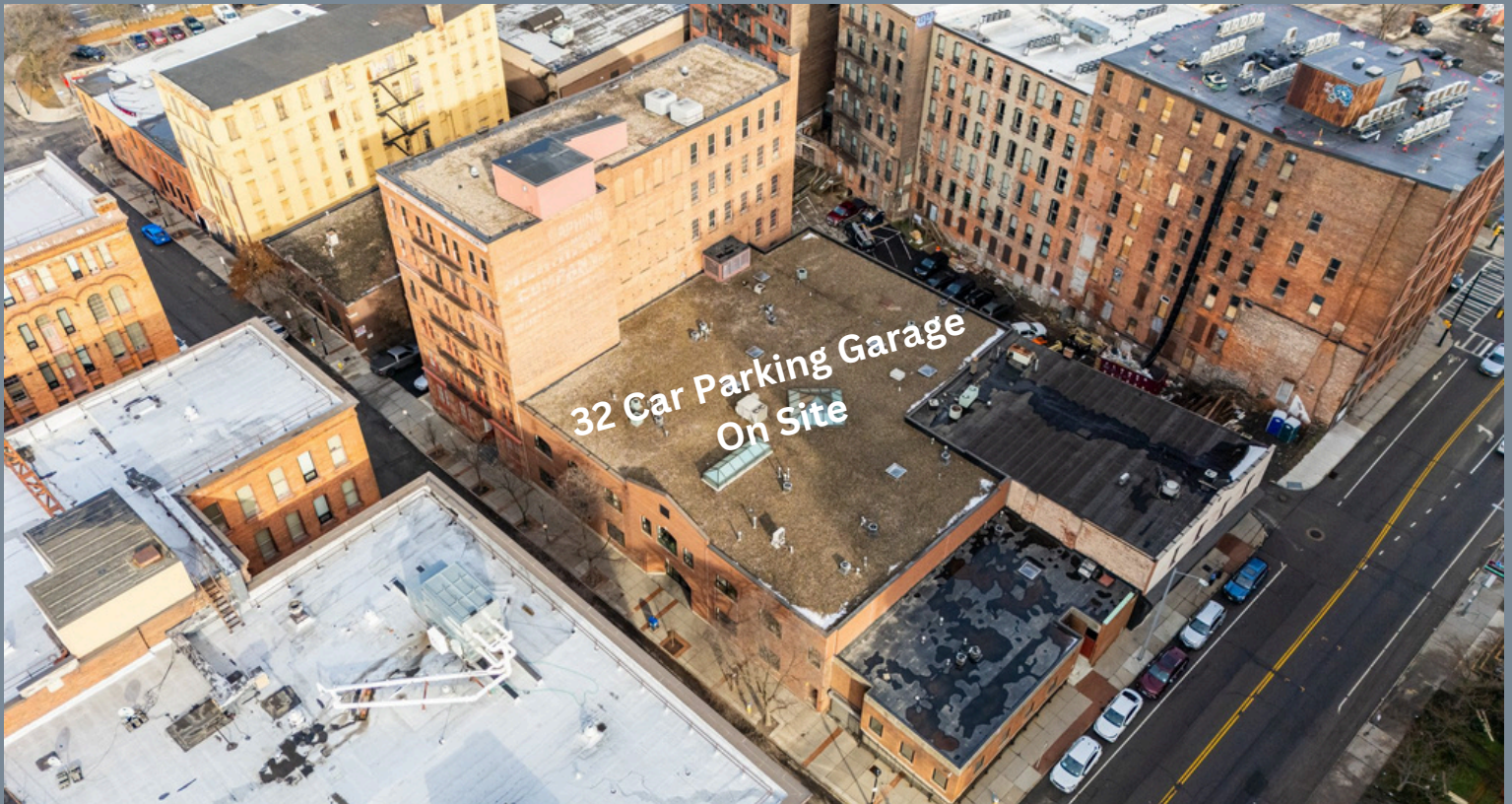
168-176 N Water Street | Rochester, NY 14608
