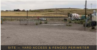
SITE — YARD ACCESS & FENCED PERIMETER
