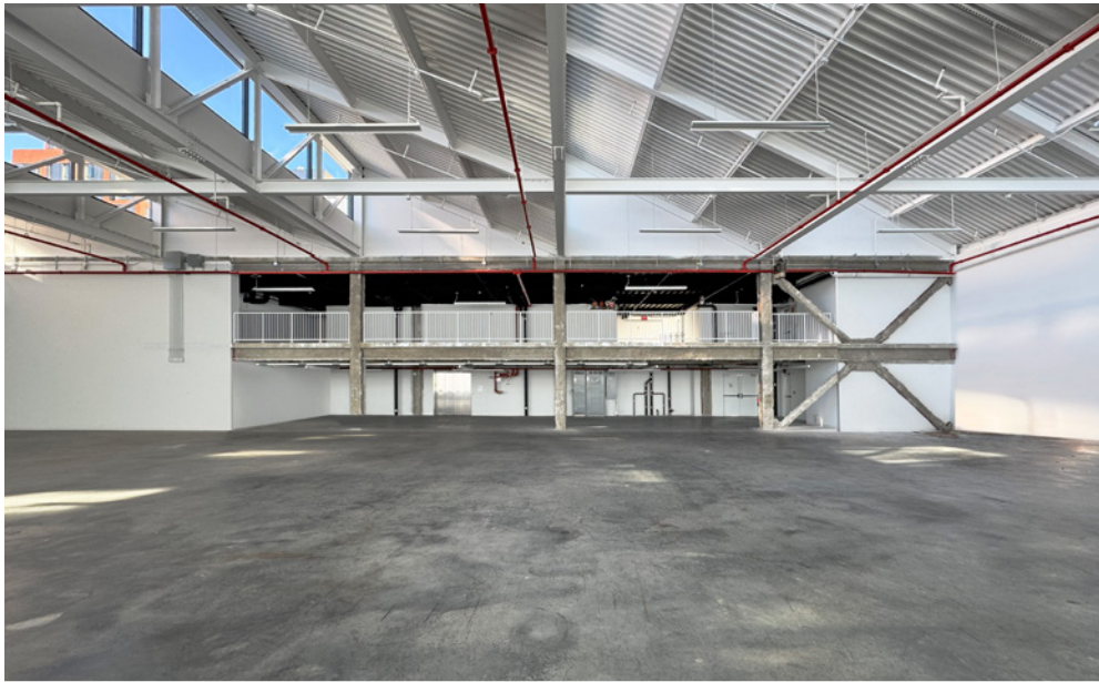
Unit 8 - View of the Mezzanine
